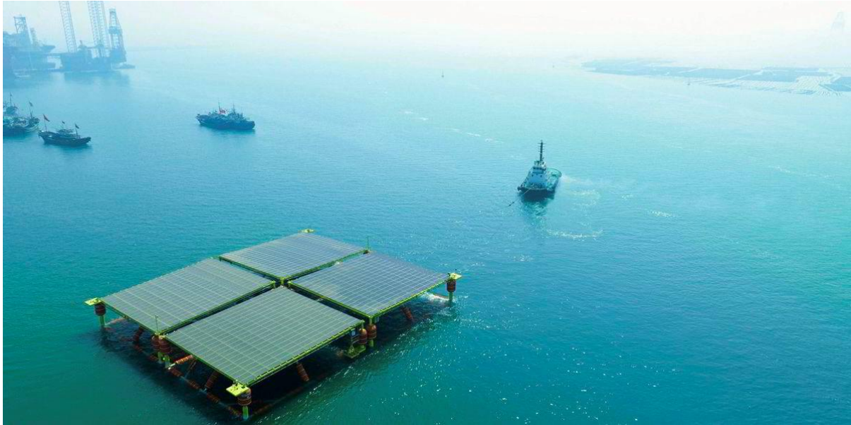
Figure 5.10.2: China's Floating Solar Power Platform at Bohai Bay (Xu, 2023)
